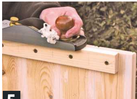
5 If panels are too tight in frame, plane relevant edges to ease fitting. Use spacers on floor to aid positioning
